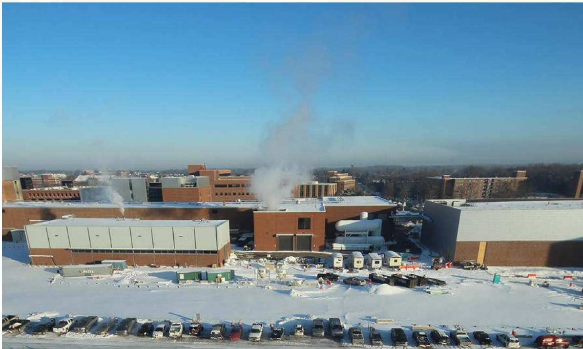
An image of site preparation currently going on at FRIB—taken by a camera mounted on the building directly to the south (facing north)
